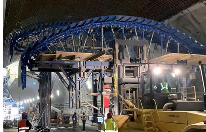
New lining – cast in place
